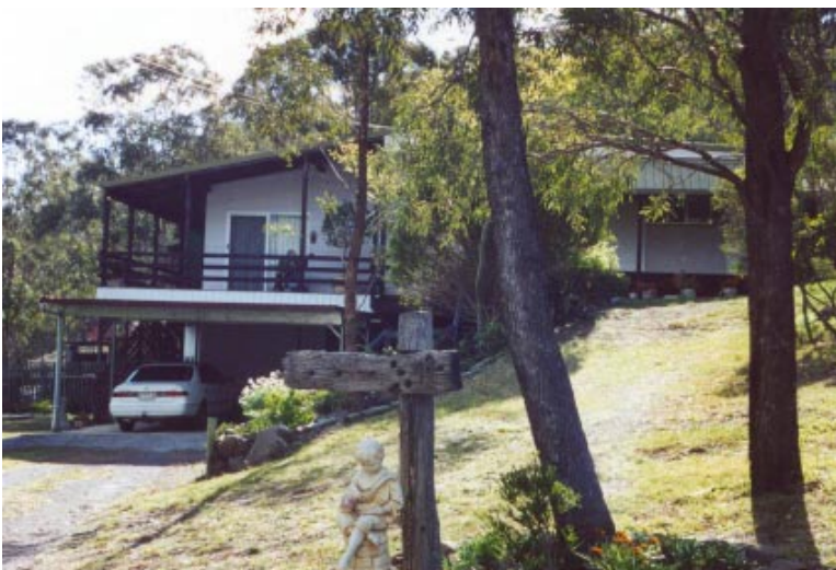
Home: The house that Rob and Wita built in Queensland.
